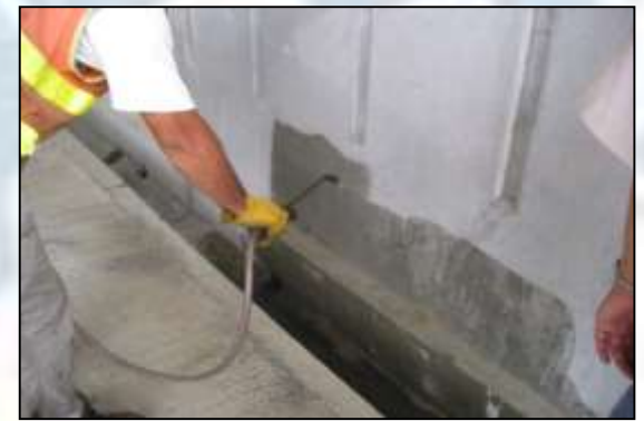
Application on the Wall
